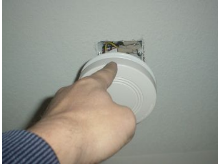
Interior Areas Smoke Detectors
