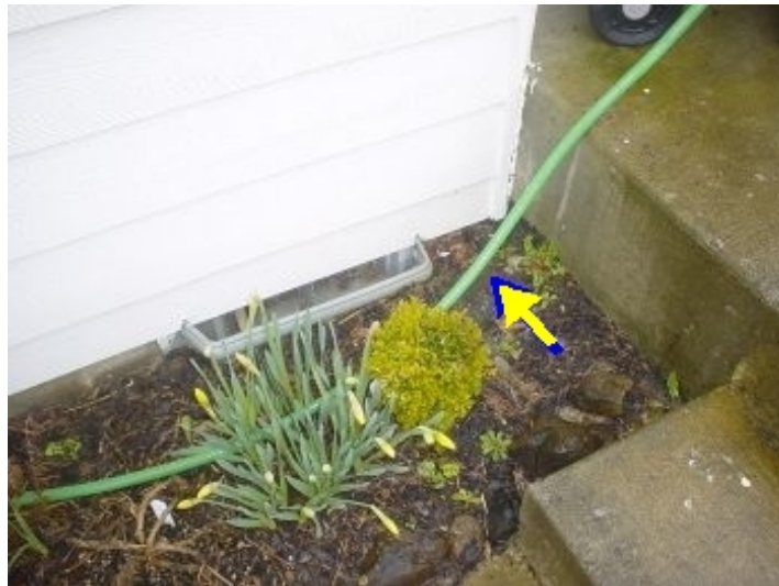
Exterior Areas Siding Condition
