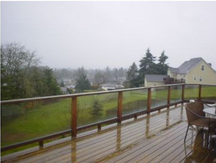
Grounds Stairs & Handrail
