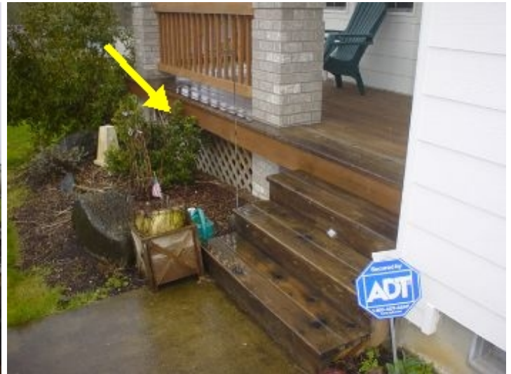
Grounds Stairs & Handrail
