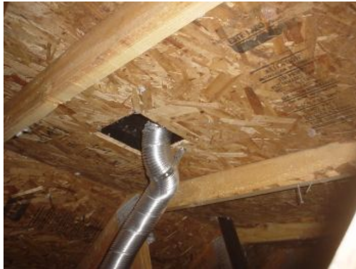
Attic Exhaust Vent
