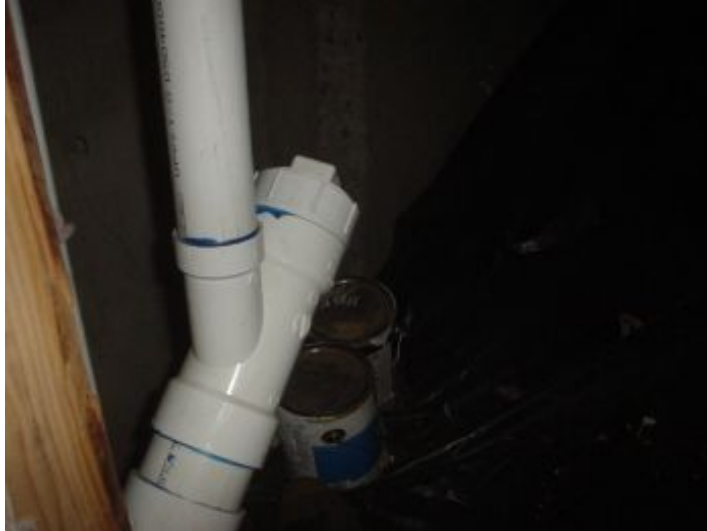
Foundation Foundation Plumbing
