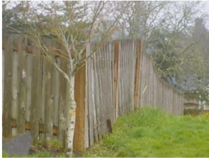
Grounds Fence Condition
