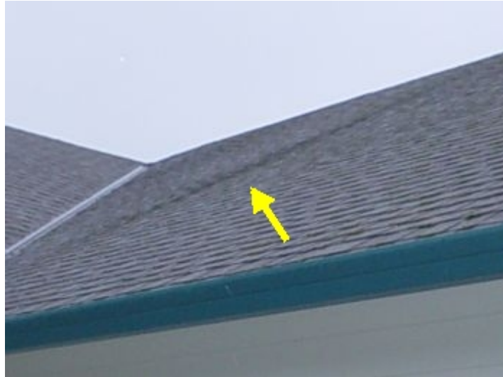
Roof Roof Condition
