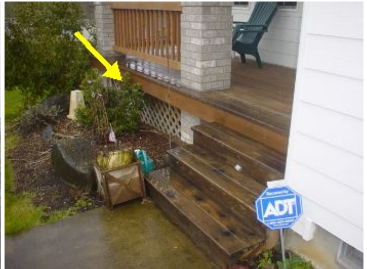
Grounds Stairs & Handrail
