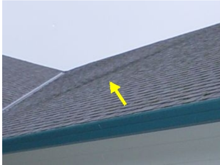
Roof Roof Condition
