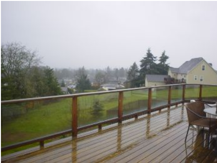
Grounds Stairs & Handrail
