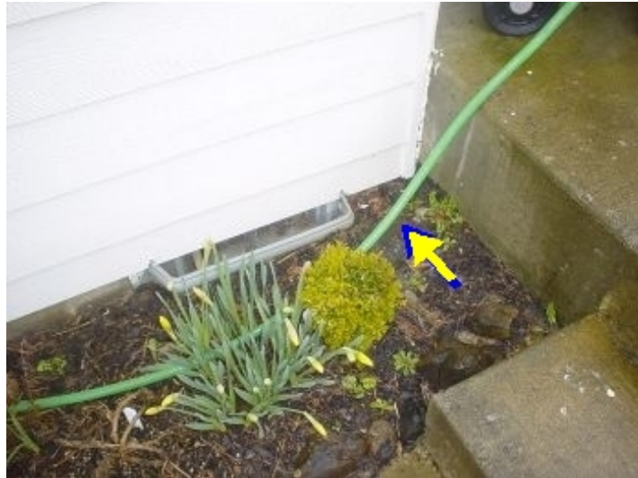
Exterior Areas Siding Condition
