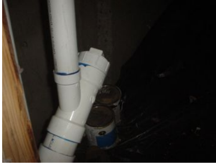
Foundation Foundation Plumbing
